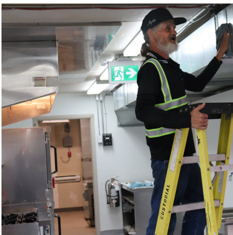
Crews from Stemic Construction working to put the finishing touches on the camp kitchen.
