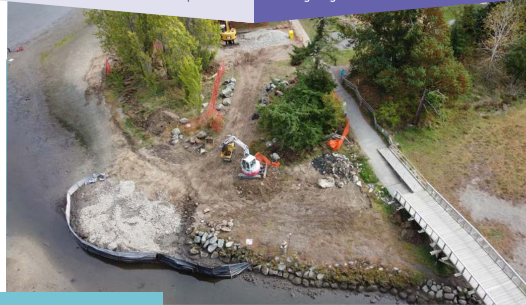
Esquimalt used Disaster Risk Reduction-Climate Adaptation funds to rehabilitate a shoreline area along the Gorge waterway.
