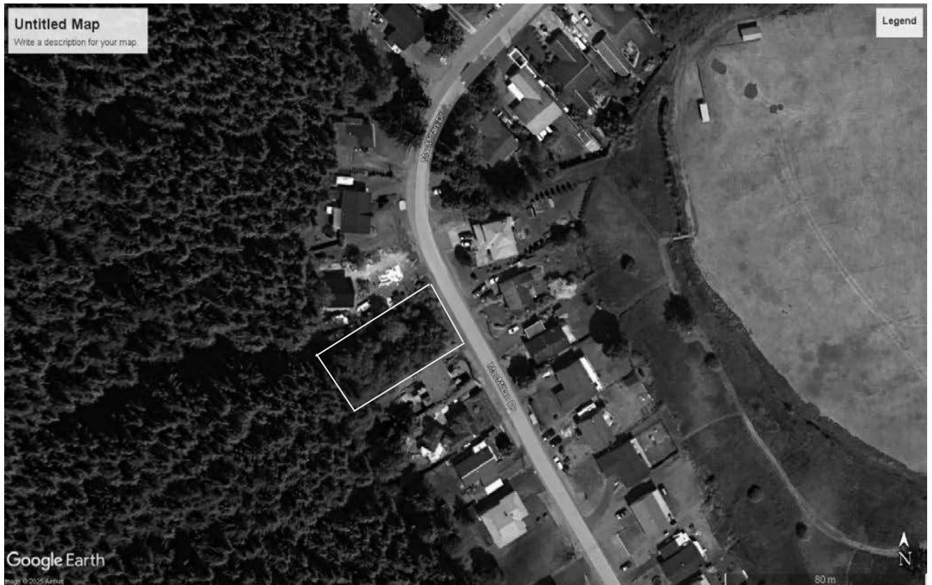
Figure 3. Google Earth imagery of 400 MacMillan Drive taken in June 2023 showing vegetation on the property. The approximate property boundary is highlighted in yellow.
