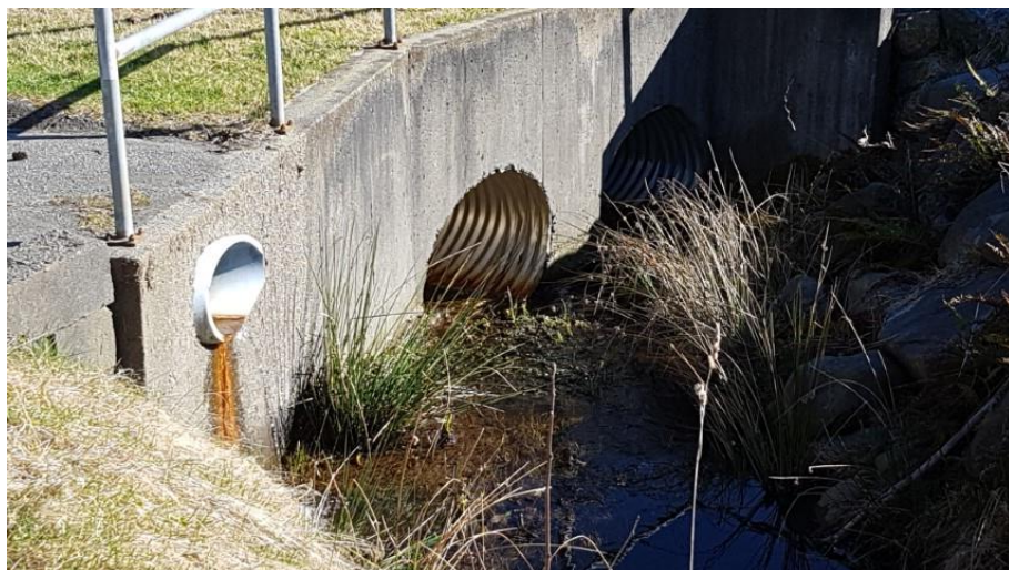
Photo 14 - Double 900mm CSP Pipe Arch Crossing of Kelsey Way
