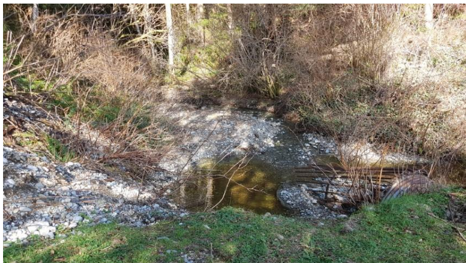
Photo 11 - Creek 3C inlet pipe/trashrack
