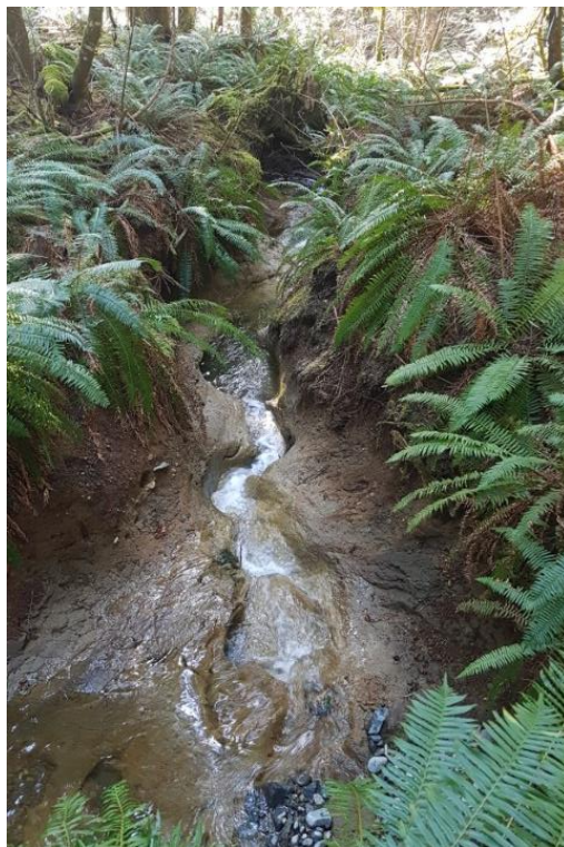
Photo 6 - Creek 3A & 3B drainage channel below wooden log diversion structure. Note exposed gravels in walls and continued erosion in bottom of channel
