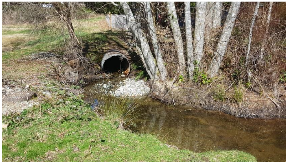
Photo 13 - Creek 3C outlet pipe at H'Kusum Park. Note pile of dredged gravels on left side of ditch.
