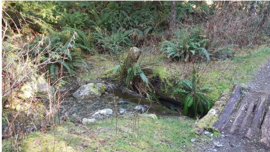
Photo 5 - Wooden log diversion structure for Creek 3A & 3B flows (water flows left to right under the trail)
