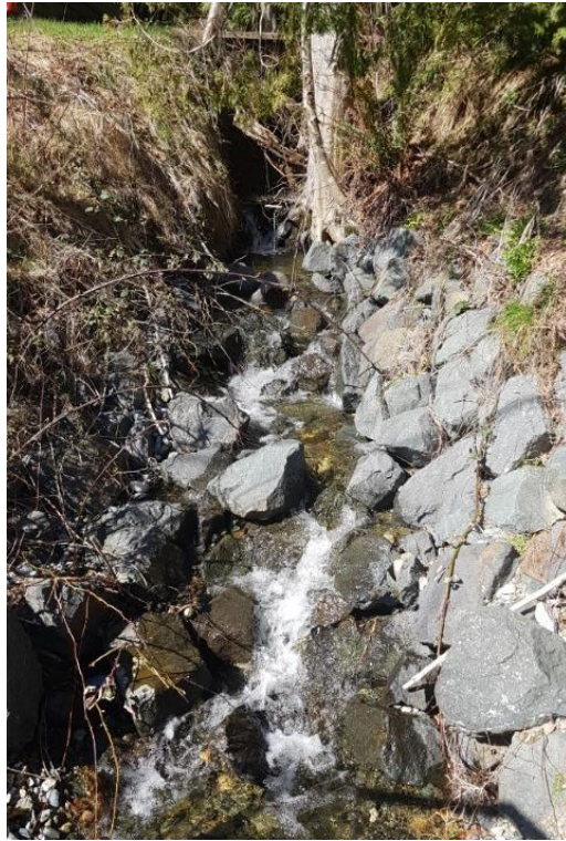
Photo 7 - Drainage ditch upstream of Headwall 1
