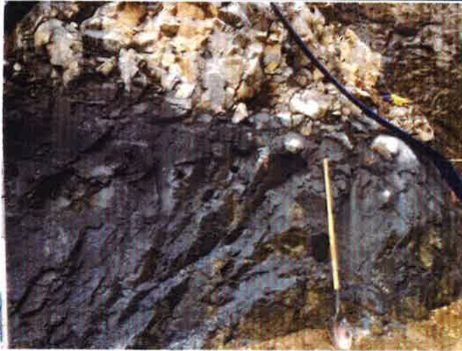
Photo 1. Footing anchor holes drilled into bedrock along the left bank at 0.5 m spacing and 2 m deep.
