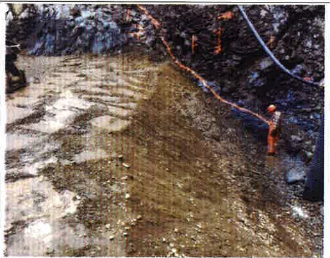
Photo 6. Completed downstream slope for cut off wall liner.
