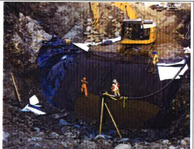
Photo 10. Partial installation of geofabric, pitrun backfill and trimming of the right side of liner.
