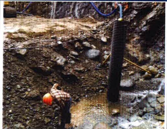
Photo 2. Cutoff trench excavated to El. 67.0. Downstream slopes is rough and being prepped for liner installation
