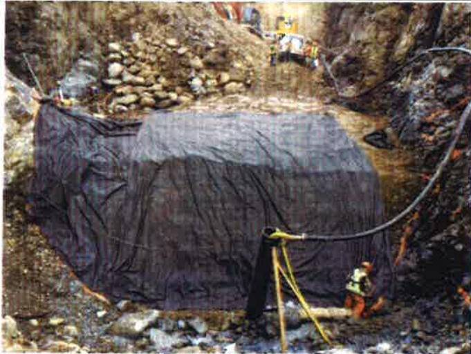
Photo 5. Geofabric installation viewed from the cofferdam
