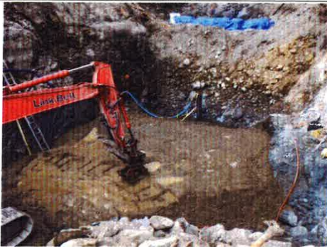
Photo 5. Excavator compacting subgrade for weir with packing attachment
