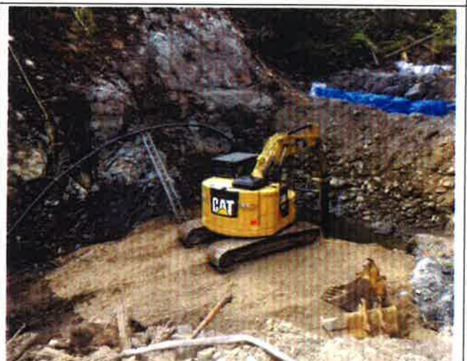
Photo 4. Cutoff wall trench water bypass hung along left bank canyon wall.
