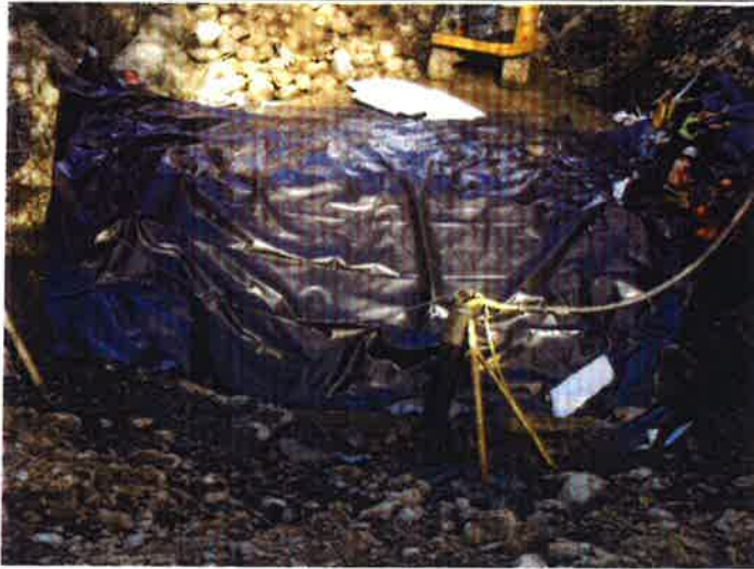
Photo 9. Liner roughly laid in trench and left side being trimmed.
