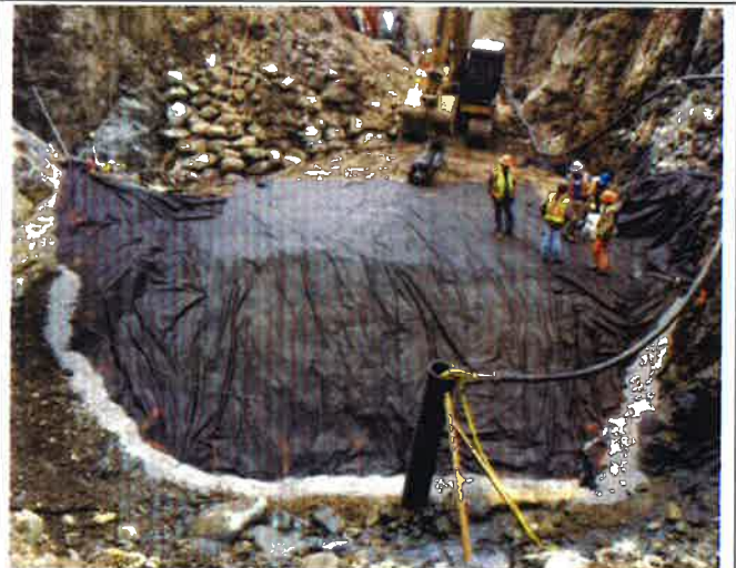
Photo 6. Bentonite pellets installed along the edge of geofabric. Full extent not completed to allow for folding back liners for form work.
