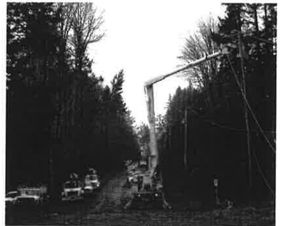
Crews repairing extensive damage in Nanaimo.
