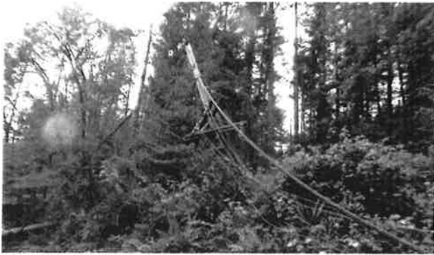
Example of infrastructure damage on Gabriola Island.
