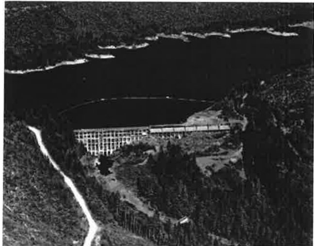
Jordan River Diversion Dam and Reservoir.
