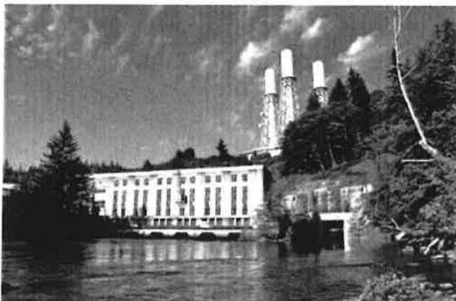
View from Campbell River of the tailrace tunnel outlet to the right of the old generating station.
